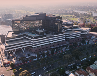
Footscray Hospital Multiplex
