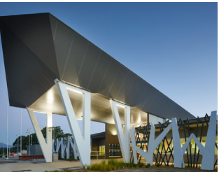
Hopkins Correctional Centre Multiplex
