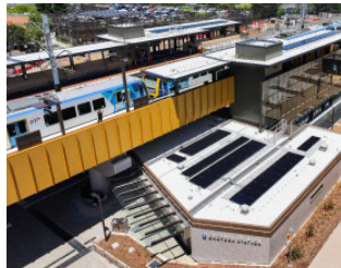
Croydon Station SEPA
