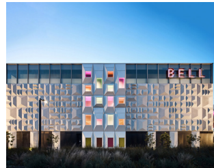
Bell Station NWPB
