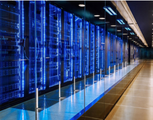
MEL060 ROMP02 Hutchinson Builders
