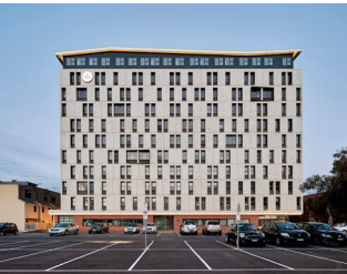
Deakin University Geelong L.U. Simon Builders
